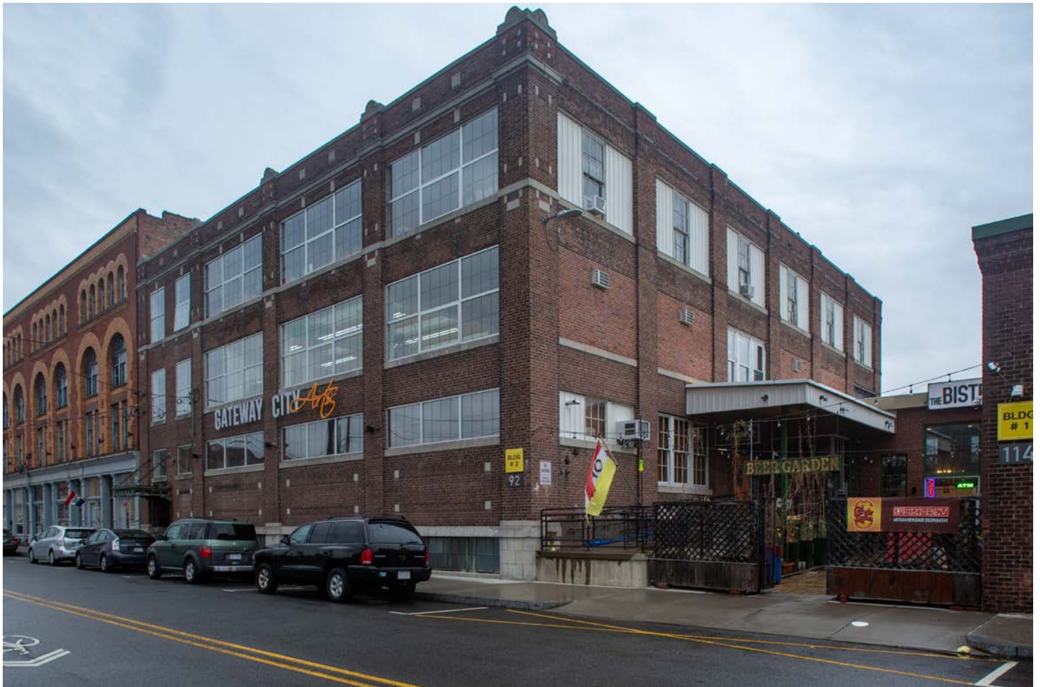
View from the southeast showing the south elevation. Photo by Zachary Violette
